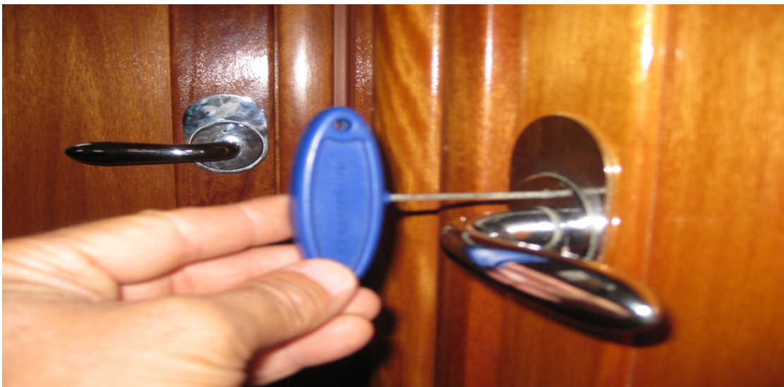
By pressing the key into the top hole of the door mechanism, you unlock the door.
